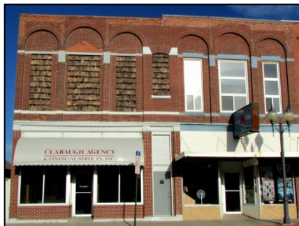
Upper-level windows and 1 st floor storefronts are in need of restoration.
