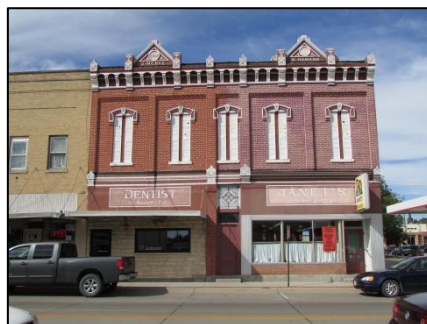
Upper-level windows and 1 st floor storefronts are in need of restoration.
